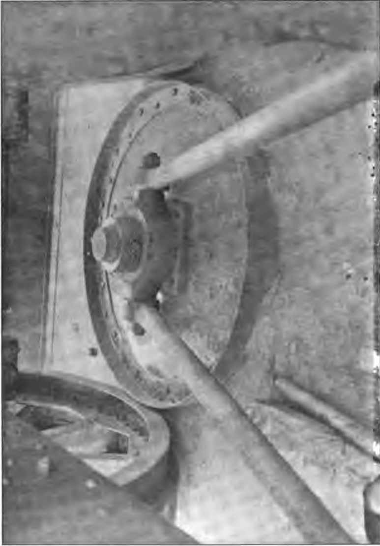
CENTER PIVOT AND TENSION RODS OF THE 170 MM. GERMAN GUN MOUNT.
